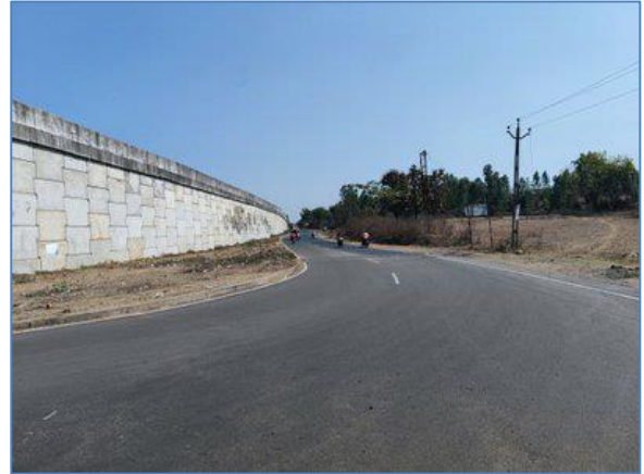
Service Road @ km 162.340 to km 163.200- RHS_7m wide
