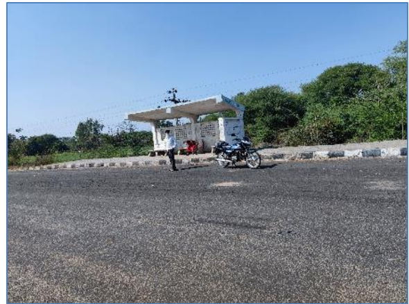
Bus Bay with shelter near km 160.080, LHS Main Carriageway
