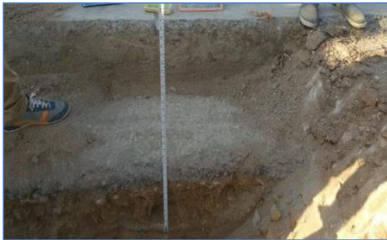
km 134.950 RHS (GMP-TP-2)
