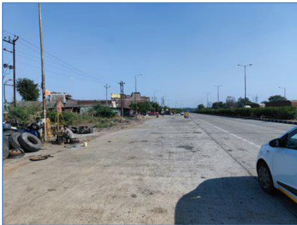
Truck Lay bye on LHS km 190.500
