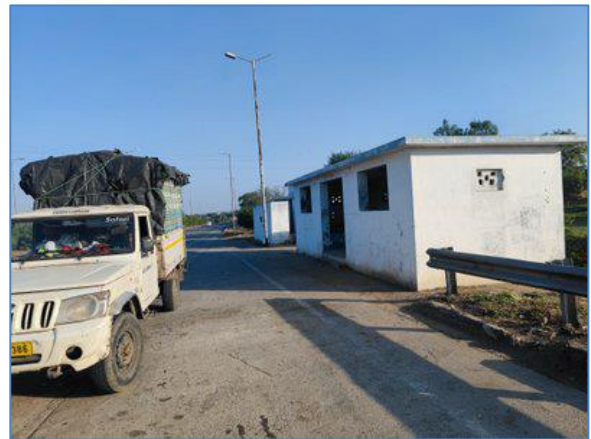
Rest Room at Truck Lay bye on RHS km 190.500
