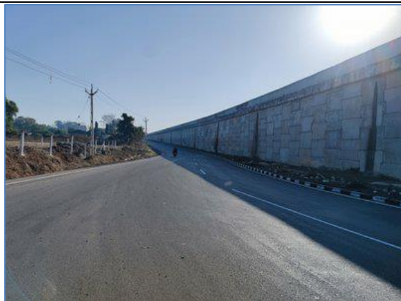
Service Road @ km 128.030 to km 128.800-LHS_7m wide
