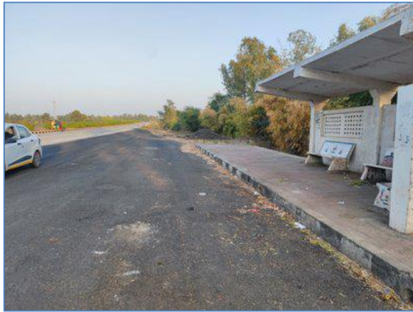
Bus bay with shelter near km 166.600, RHS Main Carriage way
