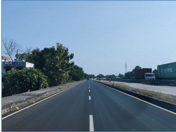
Service Road @ km 143.440 to km 144.260- LHS_5.5m wide
