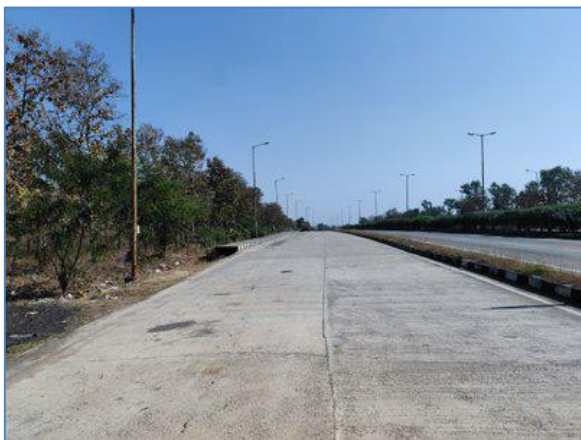
Truck Lay bye on LHS km 134.400
