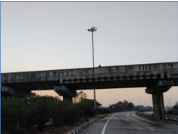
High mast lighting on Island at overpass location at km 153.720
