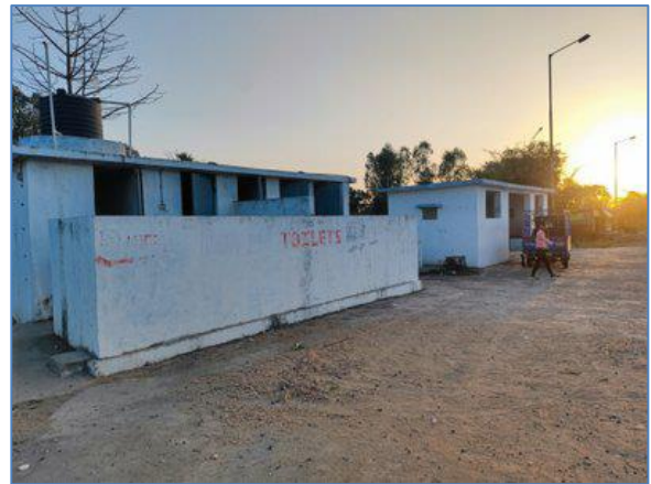
Toilet Block and Rest Room at Truck Lay bye on RHS km 157.800
