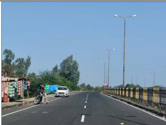
Service Road @ km 173.600 to km 174.210- LHS_7.5m wide
