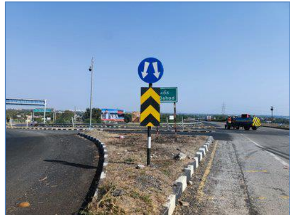
Towards Dahod town at km 189.450 (junction)
