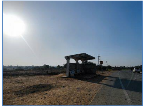
Bus shelter near km 201.400, RHS Main Carriage way
