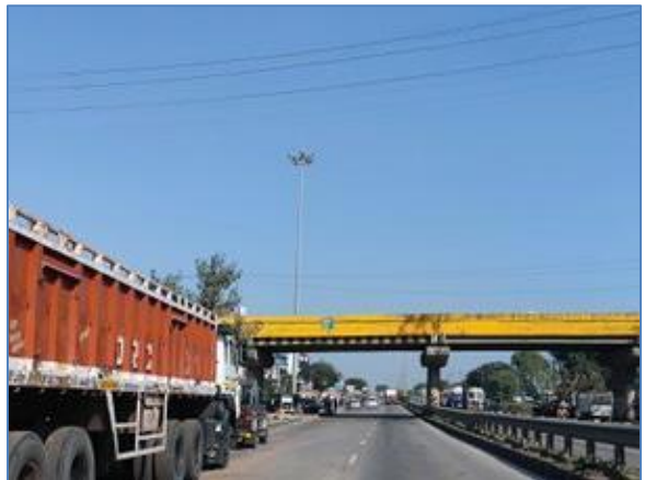
High mast lighting on Island at overpass location at km 193+800
