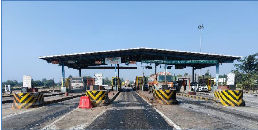
Toll Plaza near km 146.150
