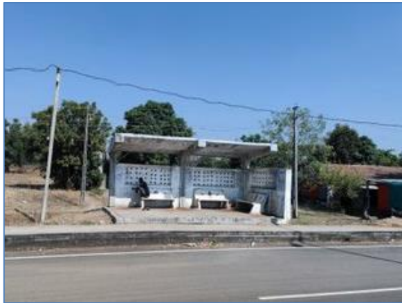
Bus Shelter near km 131.780, LHS Service Road
