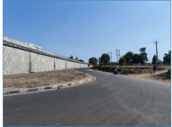
Service Road @ km 151.700 to km 152.400-LHS_7m wide
