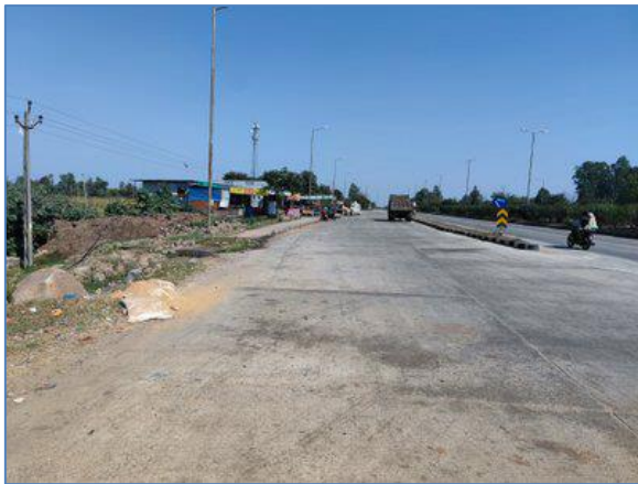
Truck Lay bye on LHS km 157.800
