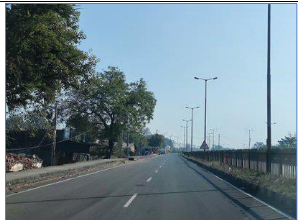
Service Road @ km 131.610 to km 132.090 LHS_7.5m wide
