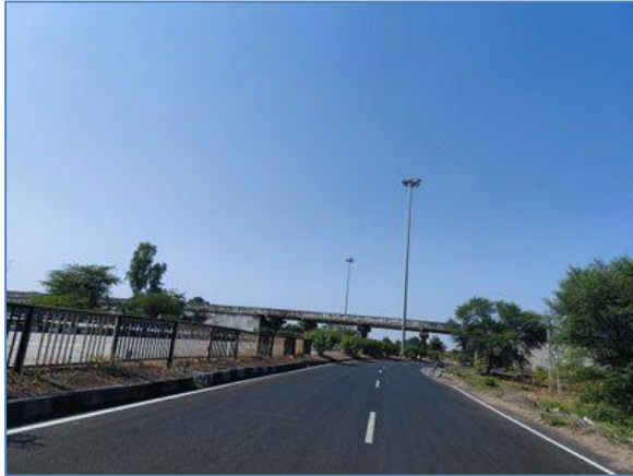
Service Road @ km 153.520 to km 153.620- LHS_5.5m wide
