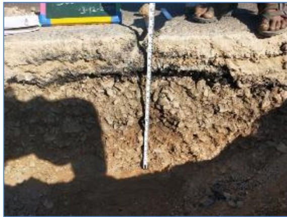
km 355+600 RHS (JP-TP-9)
