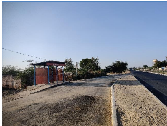
Bus Bay With Shelter near km : 336+450, RHS MC
