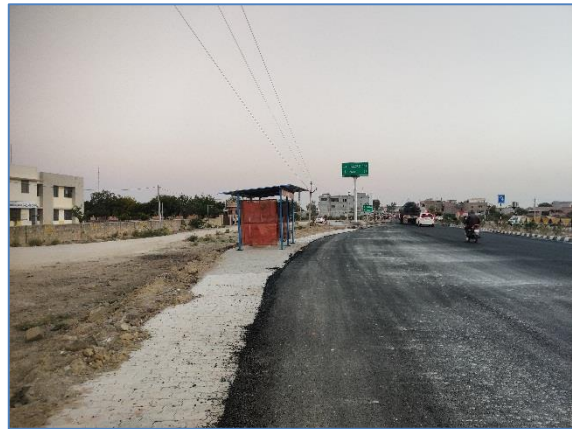
Bus Bay with Shelter near km 346.500, LHS
