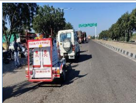
Deflection Measurement in progress
