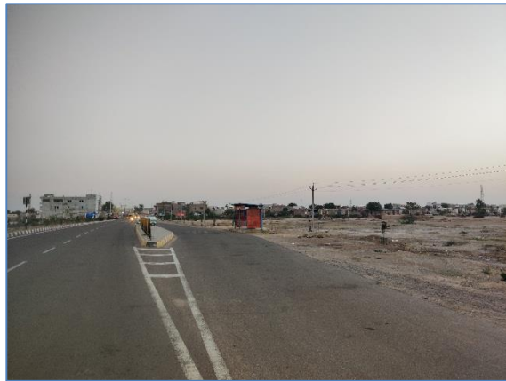
Bus shelter near km 346+450, RHS
