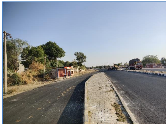
Bus Bay With Shelter near km 336+500, LHS MC
