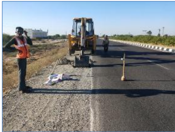
km 345+000 RHS (JP-TP-7)
