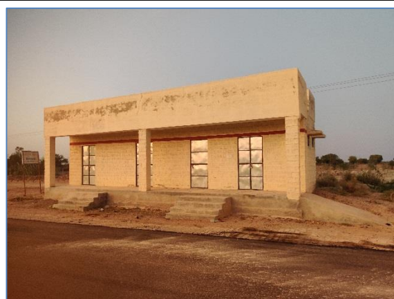
Toilet Block at Truck Lay bye on LHS km 350.400
