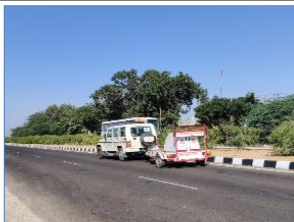
Deflection Measurement in progress
