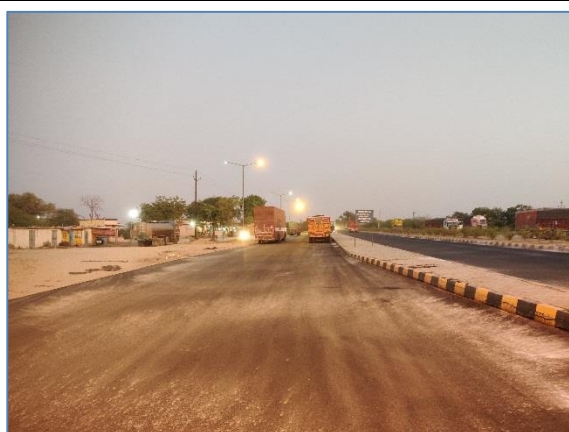
Truck Lay bye on LHS km 350.400
