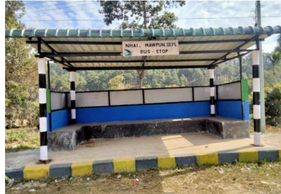
Bus Bay with Bus Shelter near km 4.450 RHS
