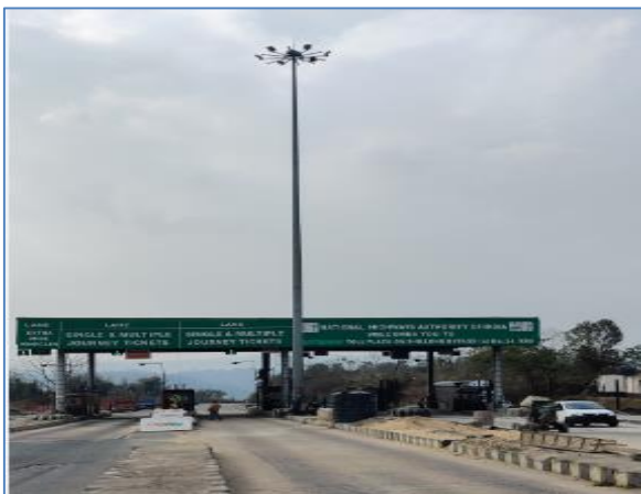
High mast lighting near km 24.900
