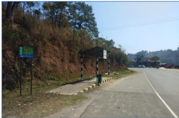
Bus Bay with Bus Shelter near km 1.500 LHS
