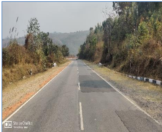
Patch work @ km 36.010
