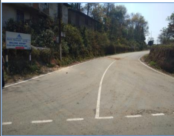
Towards Shillong Airport at km 10.130RHS
