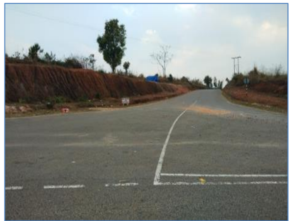
Towards Diengpasoh at km 33.530 RHS
