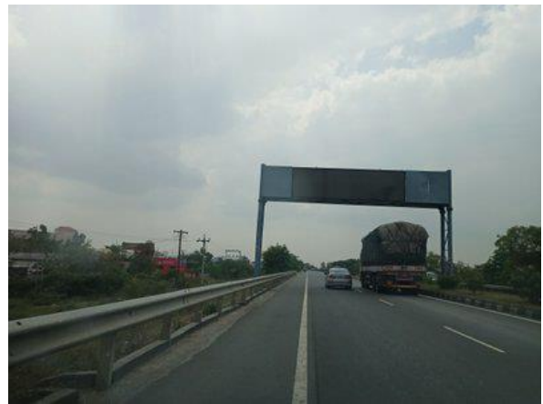
Good Condition km 165+030
