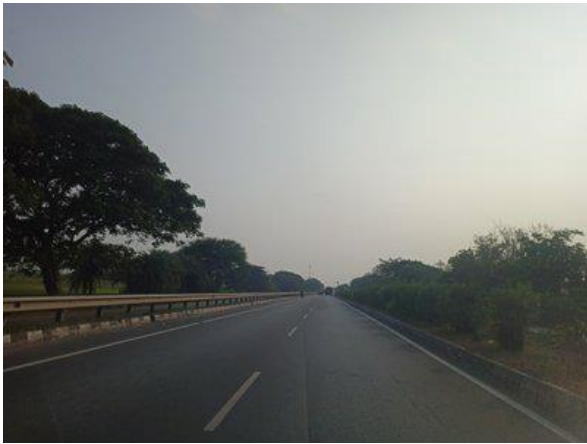
Good Condition @ km 142+450
