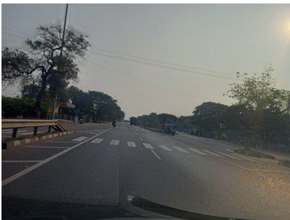
Good Condition km 144+860
