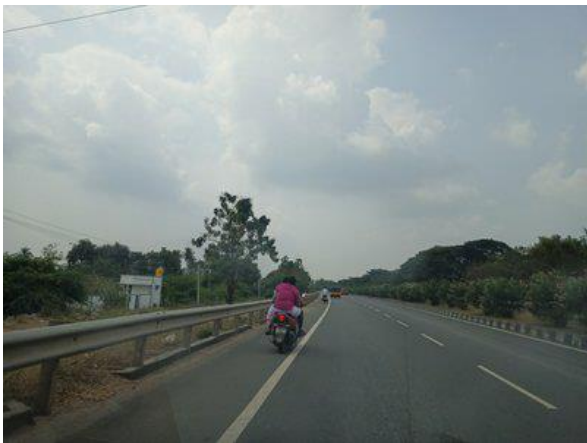
Good Condition km 161+000
