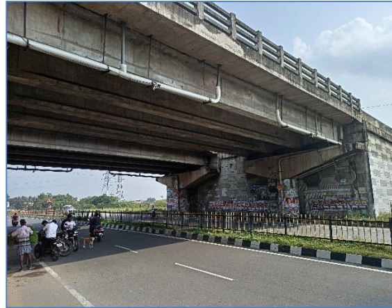
123+883 GRADE SEPERATOR (RHS)
