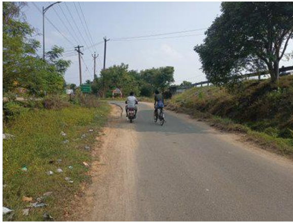
Service Road @ km 121+830-LHS_5.5m wide
