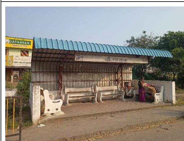
Bus Bay With Shelter @ km 150+600, RHS MCW
