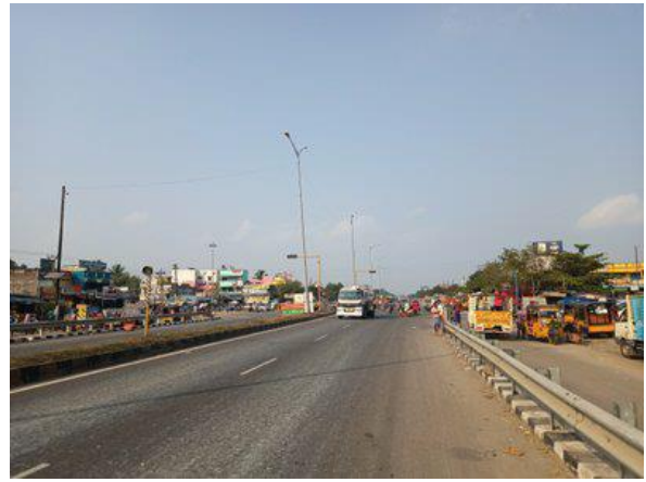
Good Condition km 133+770
