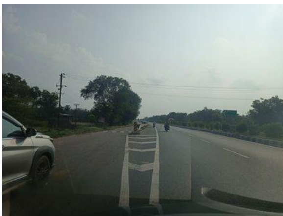
Service Road @ km 128+530-LHS_5.5m wide
