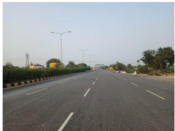
Good Condition @ km 149+880
