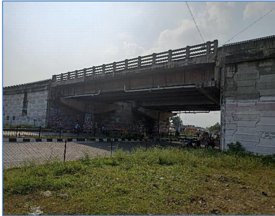
123+883 GRADE SEPERATOR (LHS)
