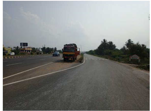
Service Road @ km 123+180-LHS_5.5m wide
