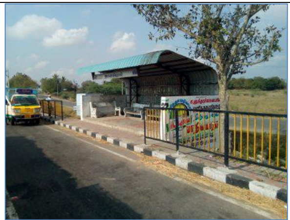
Bus Bay with Bus shelter @ km 168+100, RHS MCW
