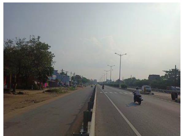
Service Road @ km 131+630-LHS_5.5m wide
