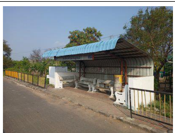
Bus Bay with Shelter @ km 131.830, RHS MCW
