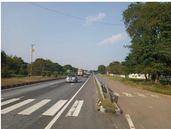
Good Condition km 128+870
