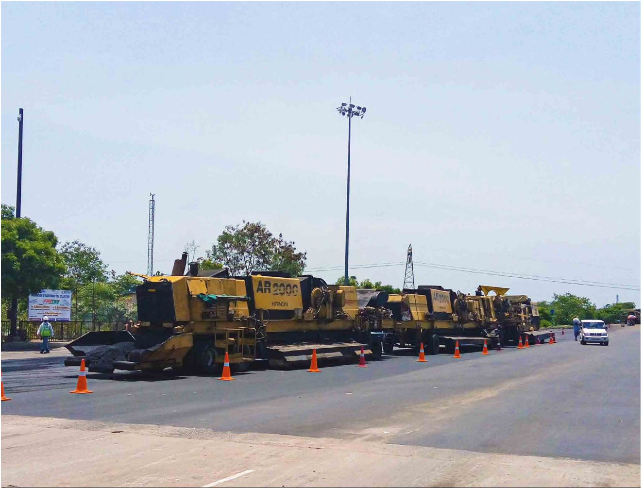
HIPR Work in Progress at UEPL Project Site
